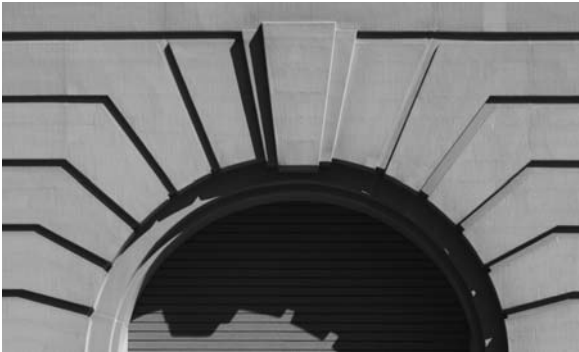
A keystone is the center stone in an arch
